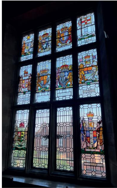
Fig.14 Photo showing existing stained glass in window.
